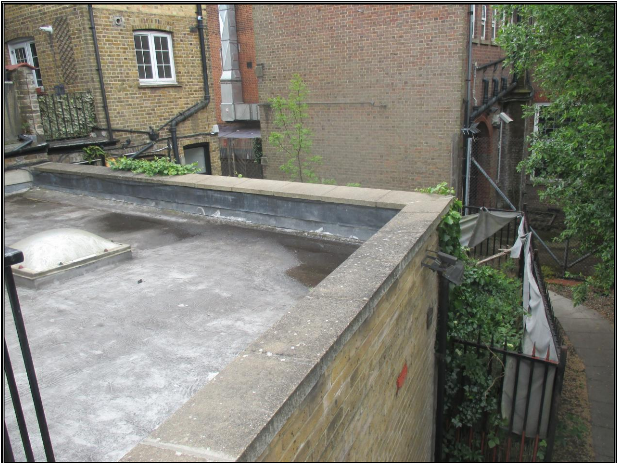
Adjoining shop showing rear extension.
